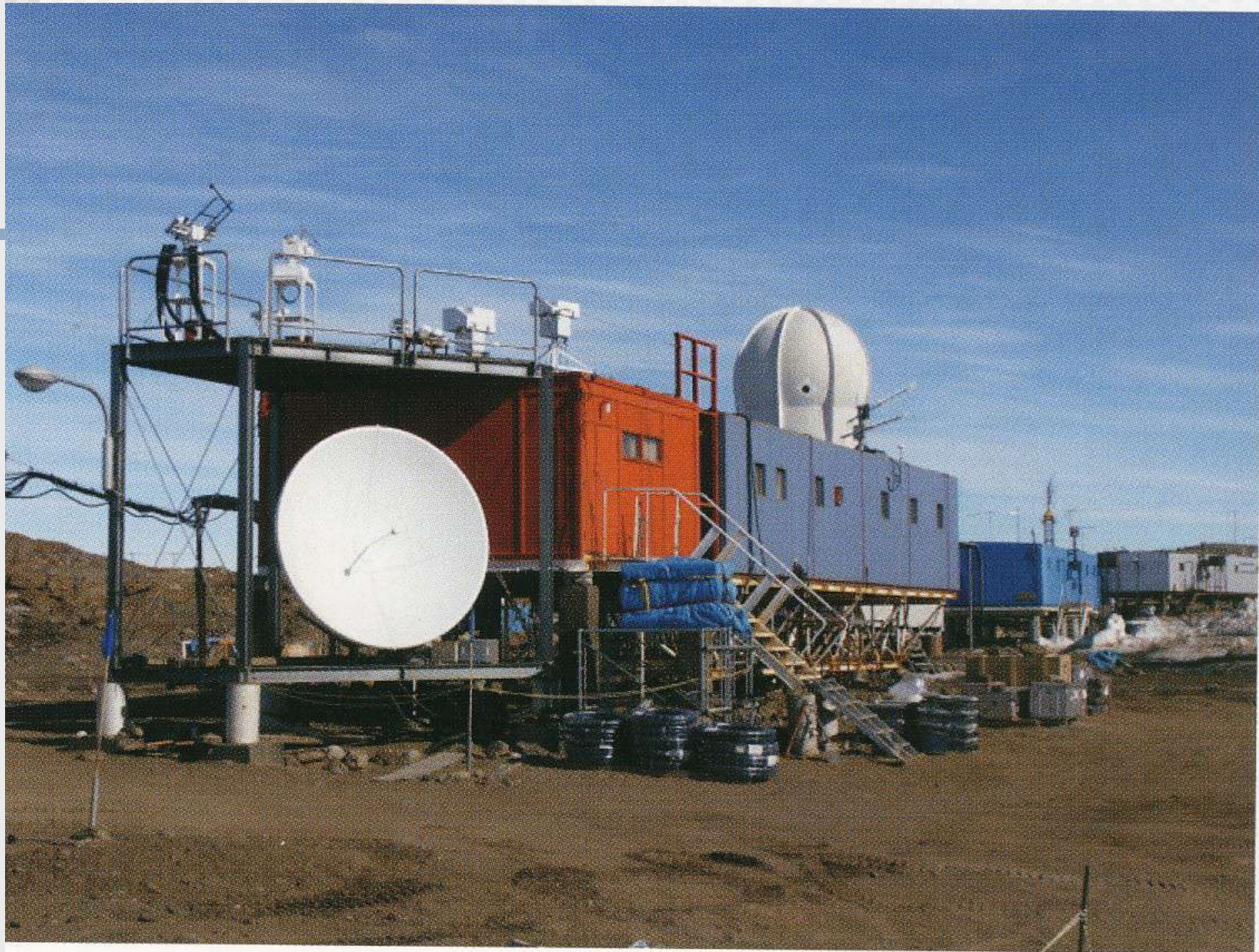
Meteorological observations hut, Syowa station
