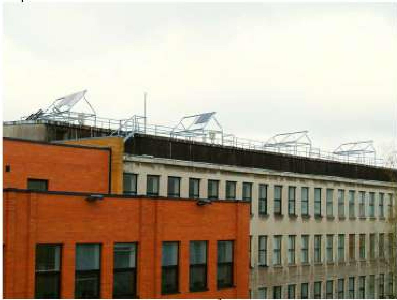
Figure 1. Four metal frames for mounting of up to 32 m<sup>2</sup> of modules on the roof of Material Science department
